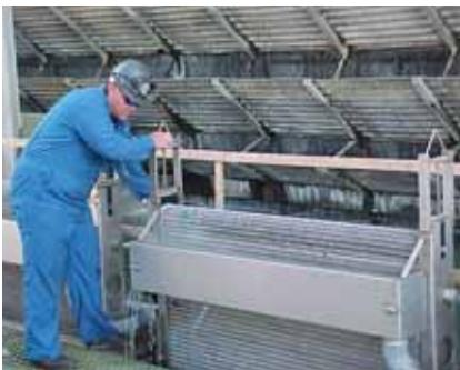
Traveling sump screens are designed to capture debris before it reaches the pump.
